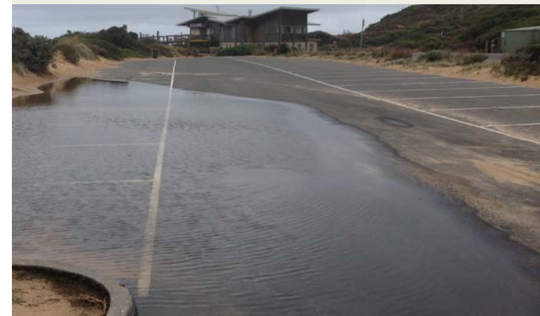
Wind blown sand into the car park has created ongoing problems. This includes blocking of stormwater drains and the need for regular removal of the sand deposits from the car park area.
