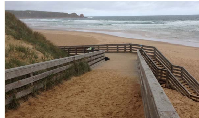
The existing ramp and stairs leading to Woolamai Beach are used by visitors, recreational users and the Surf Life Saving Club for their life saving equipment and beach rescue vehicles.
