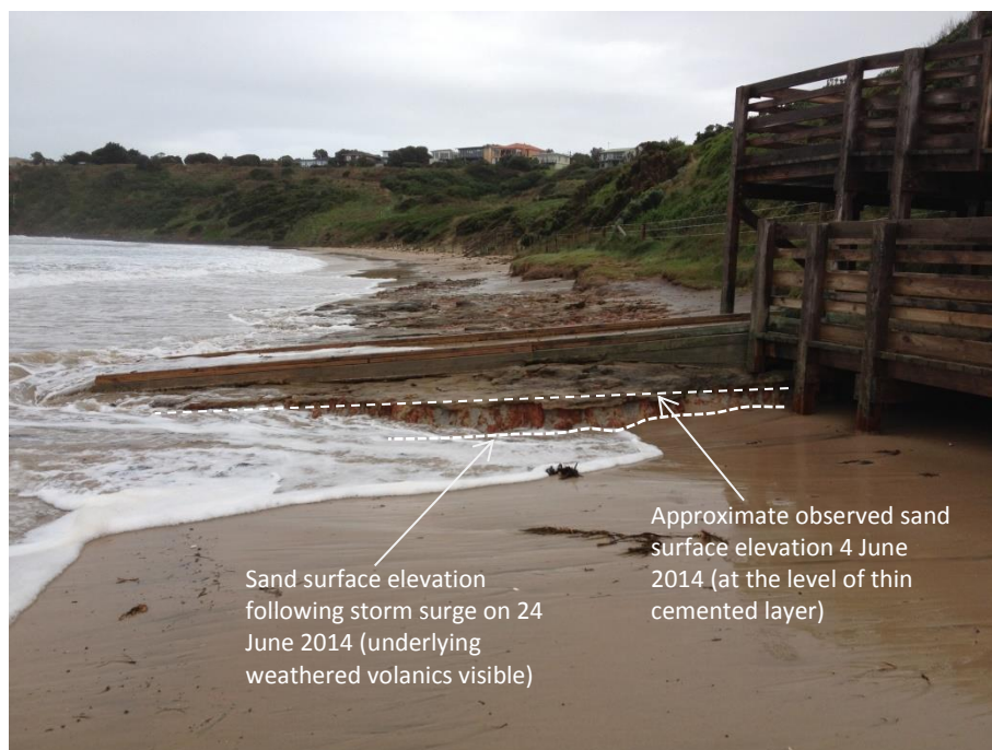
Figure 3-6 Interface between the beach and backshore in June 2014, following a storm surge event
