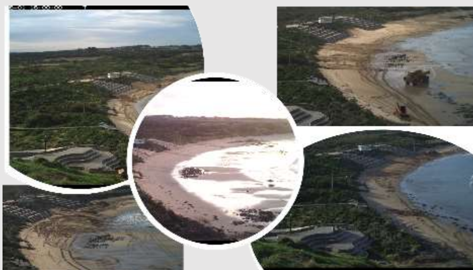
Above photos: The extensive five-day sand nourishment carried out in winter 2021 has restored the historical beach profile at the Summerland Beach.
