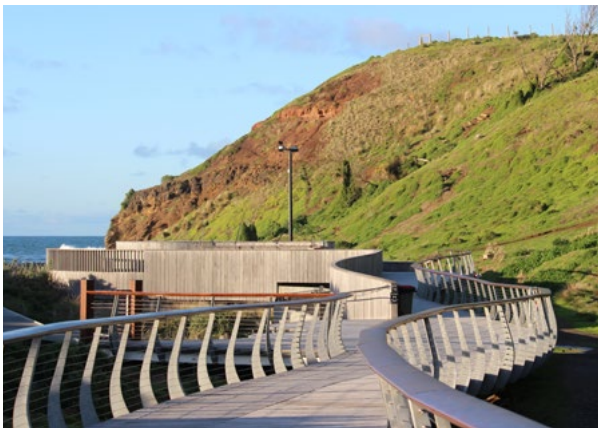
Penguins Plus viewing platform ramp access
