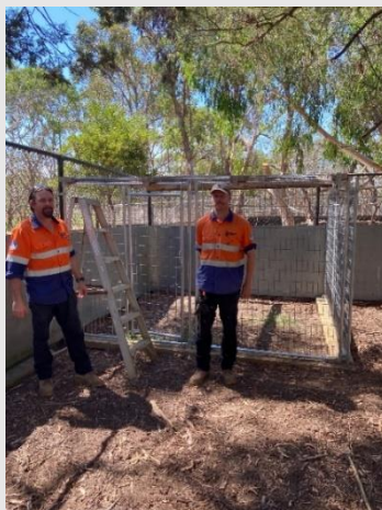
Above photo: Renovations underway at the pens to house the koalas
