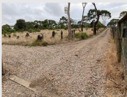
Photo: Completed new tracks
