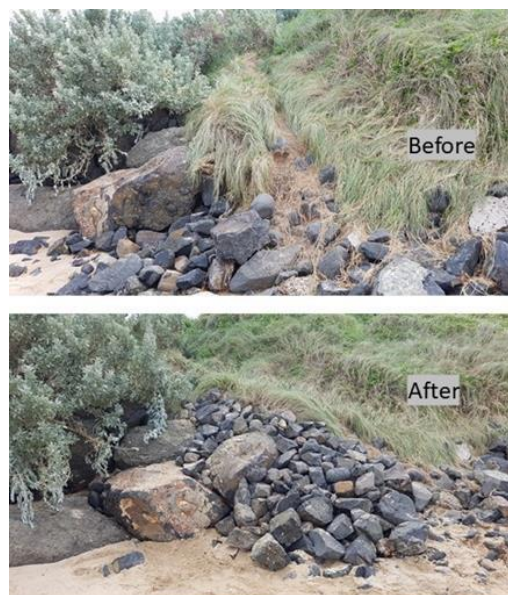
Photo - The collapsing of the penguin path between the Penguin Parade viewing standings; before and after repairs by the Visitor Experience rangers.
